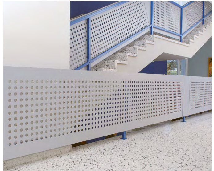
STAIR RAILING - HOLE MILLING
